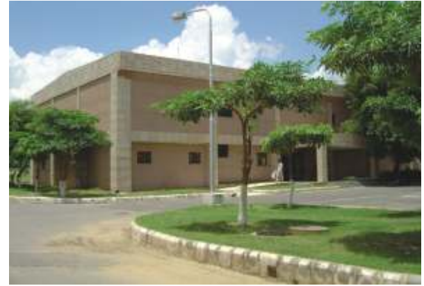
The Animal Facility Building of NBRC, which meets all the national and international standards.
